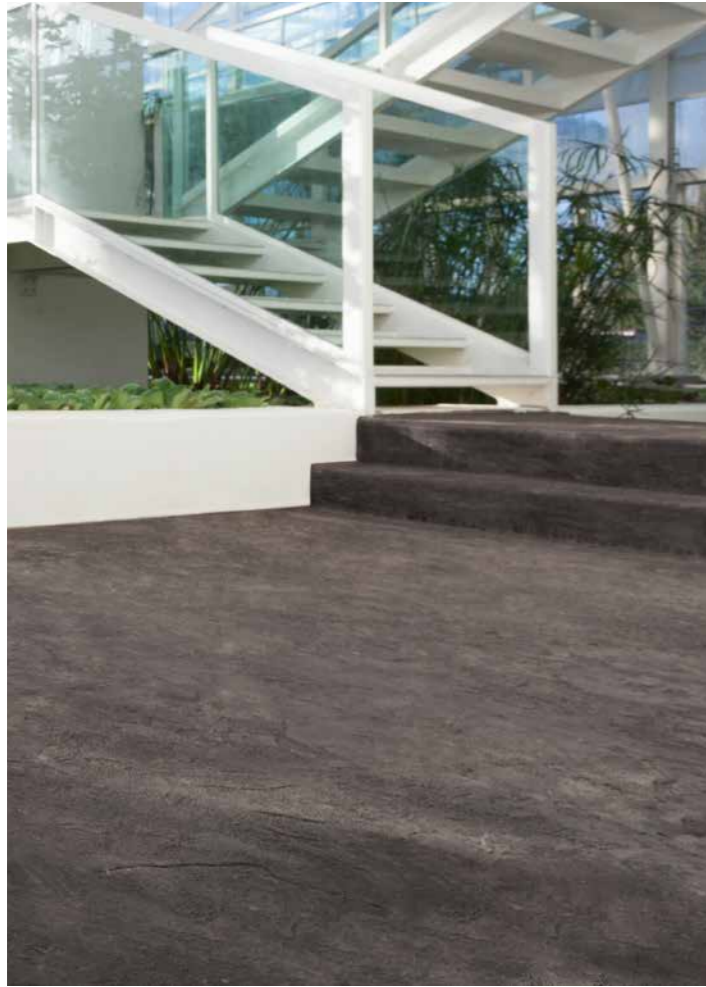
Orto Botanico 2013. Padua, Italy Stamped concrete Arch: VS Associati, Giorgio Strappazon, Fabrizio Volpato
